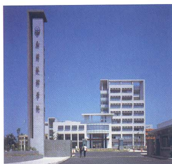
43 2001 Administration Building NanKai College
