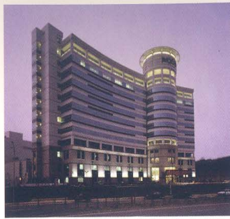
38 1999 Macronix Headquarters Building
