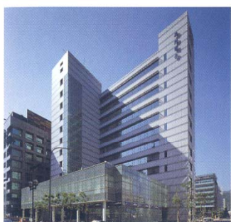
46 2002 Winbond Technology Building
